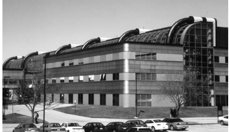
Special air supply stack systems match the atrium contour.
