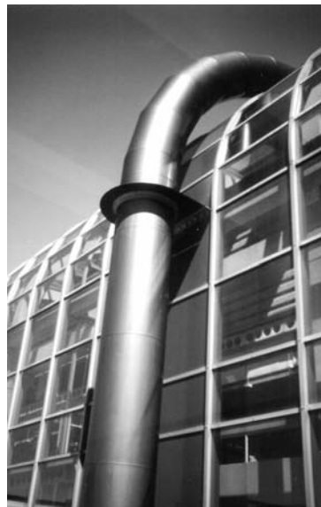
Special air supply stack systems match the atrium contour.
