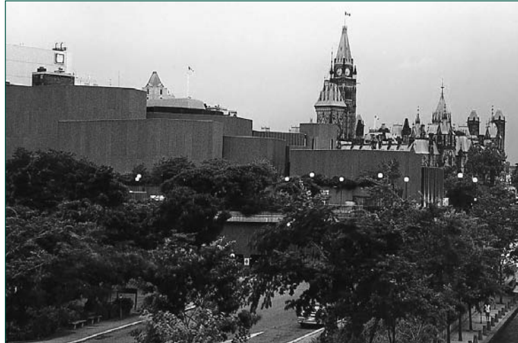
Vibro-Acoustics supplied noise and vibration products, testing and project management for the 66 fan systems and the 20 mechanical rooms for the National Arts Complex.
