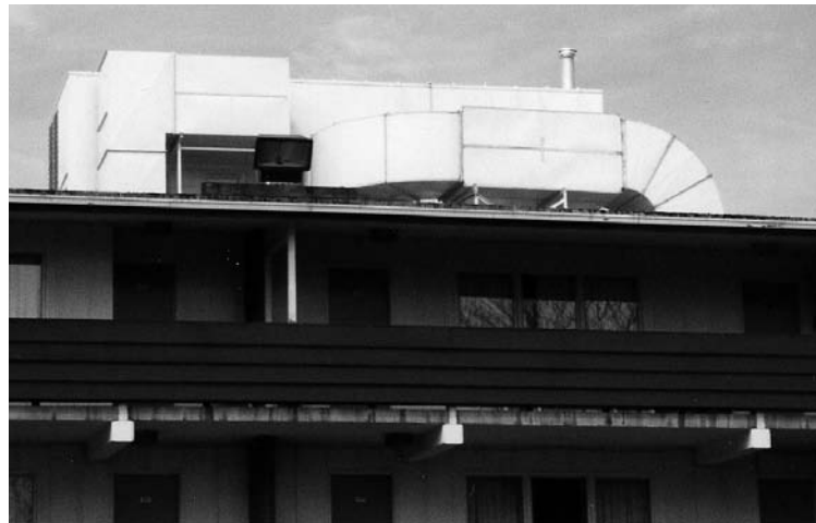
Side view of exhaust and return silencing. (Reference drawings above)
