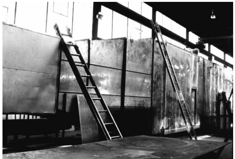
Fan / silencer package and test duct work.
