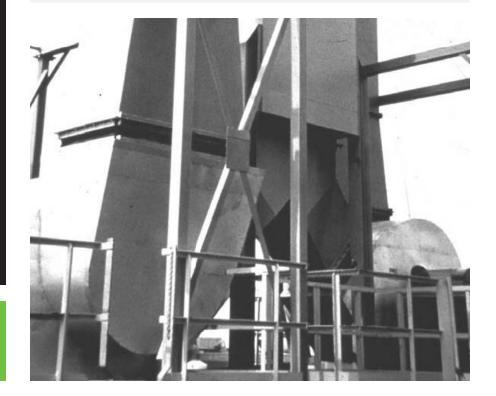
Vibro-Acoustics designed and supplied a special silencer / exhaust stack package for the 90,000 CFM tile line dust collection system.
