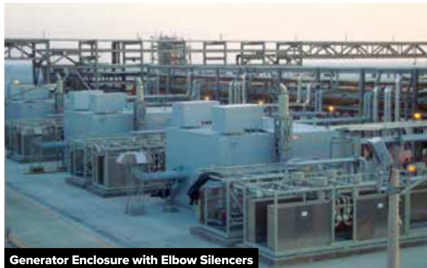
Generators with Airfoil Louvers
