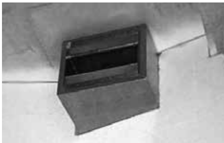
Silencer with HTL wall construction
